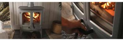
Close the door but leave it slightly ajar. This helps to heat the chimney flue for a clean burn. Once the fire is burning well close the door and reduce the air control.
